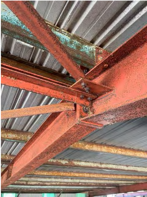
PICTURE 9 - TYPICAL RIDGE/BRACING/STRUT CONNECTION
