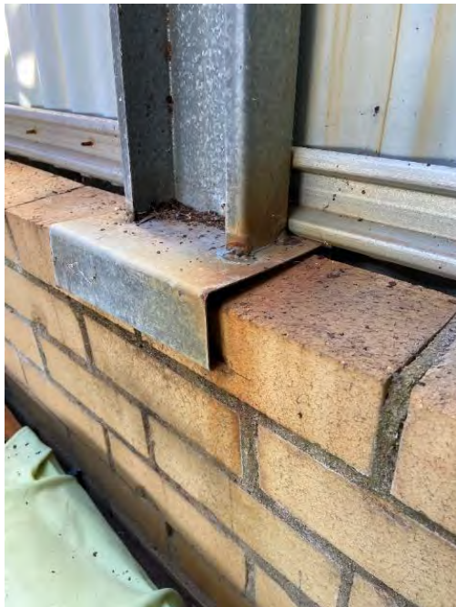
PICTURE 27 – COLUMN BASE CONNECTION
