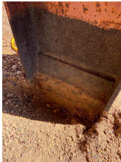
PICTURE 6 – BASE PLATE BELOW GROUND & COLUMN REINFORCEMENT
