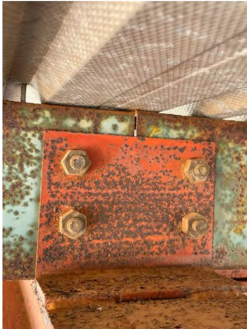
PICTURE 15 - TYPICAL PURLIN CLEATED CONNECTION
