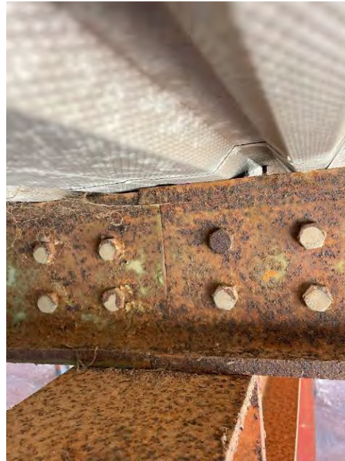
PICTURE 16- TYPICAL 'DOUBLED-UP' PURLIN CONNECTION
