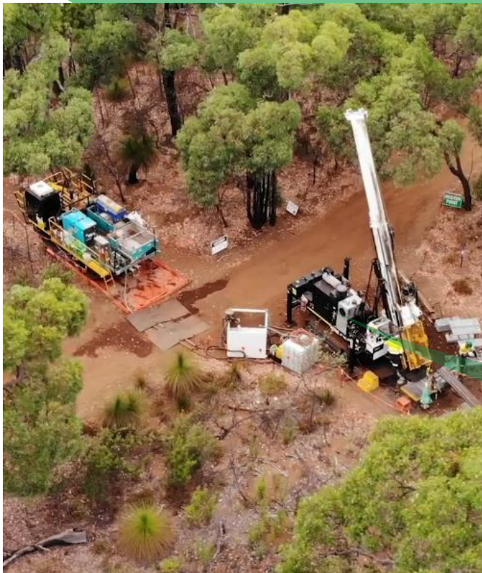
Chalice's compact drill rig operating on existing access track in the Julimar State Forest. Note: ground fluid is water, not waste fluids.
