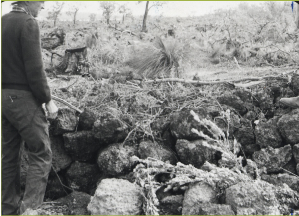
Remains of a retaining wall, made out of stones shaped and carried by convicts. Possibly these were part of the Toodyay-Guildford Road out-station
