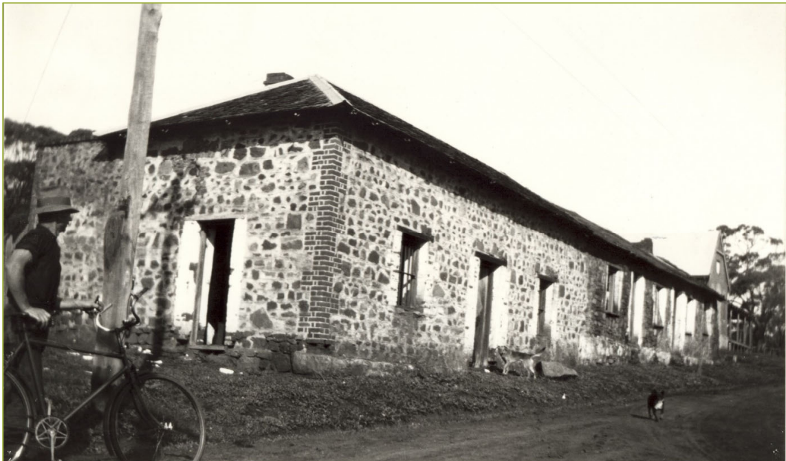
Warders' Quarters, c. 1930. The building was part of the Toodyay Convict Hiring Depot but is now demolished.
