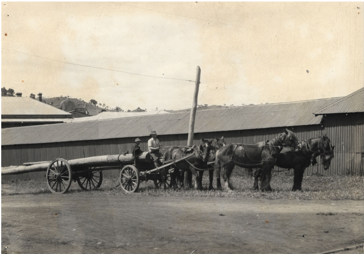
Horse drawn wagon carrying power poles, Clinton St, Toodyay, c. 1920-1930. A note on the back says "After the hole was dug, one of the team of horses was then used to maintain a forward pace as the power pole was hauled into position".
