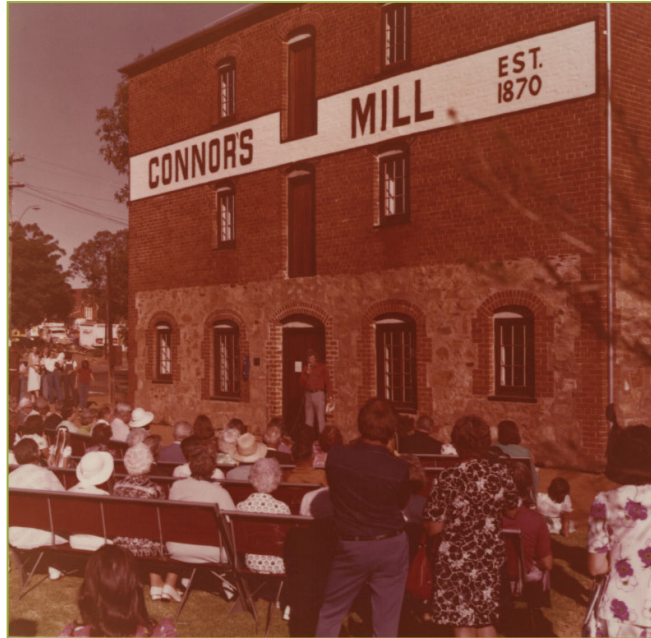
Opening of the Toodyay Tourist Centre in the refurbished Connor's Mill building, twenty years after the Road Board Power Station that was housed inside closed down.
