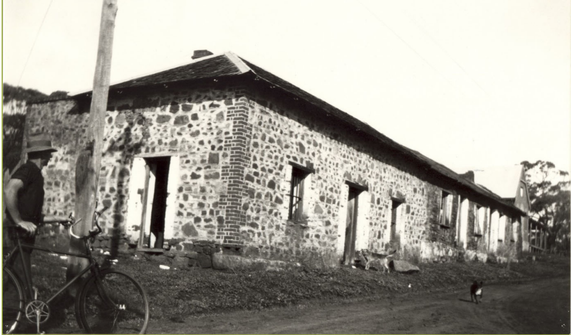
Warders' Quarters, c. 1930. The building was part of the Convict Hiring Depot but is now demolished. Shire of Toodyay local history collection 2001.1199
