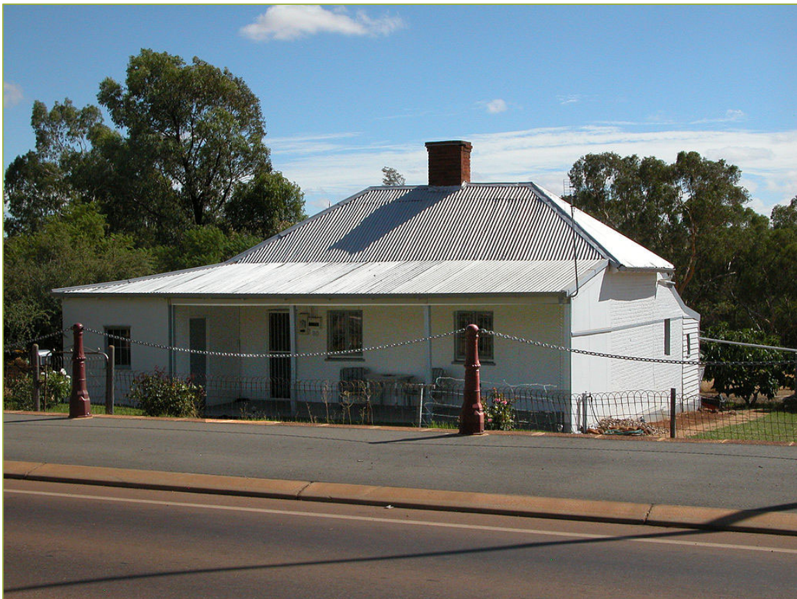
Cottage built for pensioner guard Owen Hackett. It originally had two rooms with a shingle roof that is still intact under the newer corrugated iron roofing.
